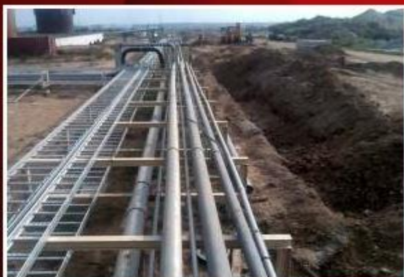
Installation of pipe sleepers and cable racks at the compressed air station at KTPP
