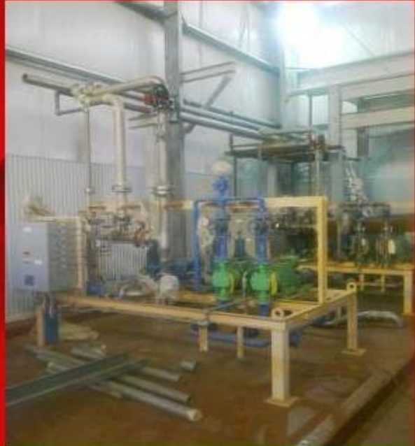
Installation Interconnecting Piping for Acid and Alkaline Regenerating Skid
