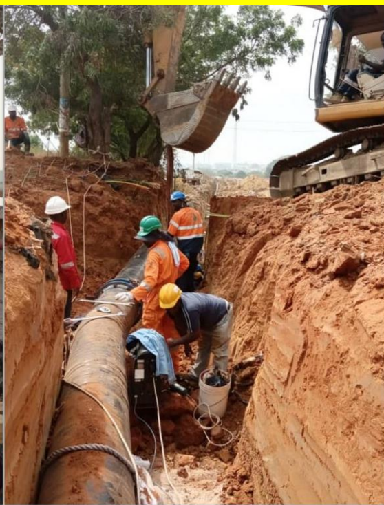
Installation of 16" LNG Pipeline from VRA Gas Interconnecting Facility to the Kpone Power Plant
