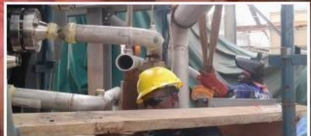
Kpone Thermal Power Project KTPP 1 Installation of fuel-gas piping from fuel-gas skid to the auxiliary block of Gas Turbine 2
