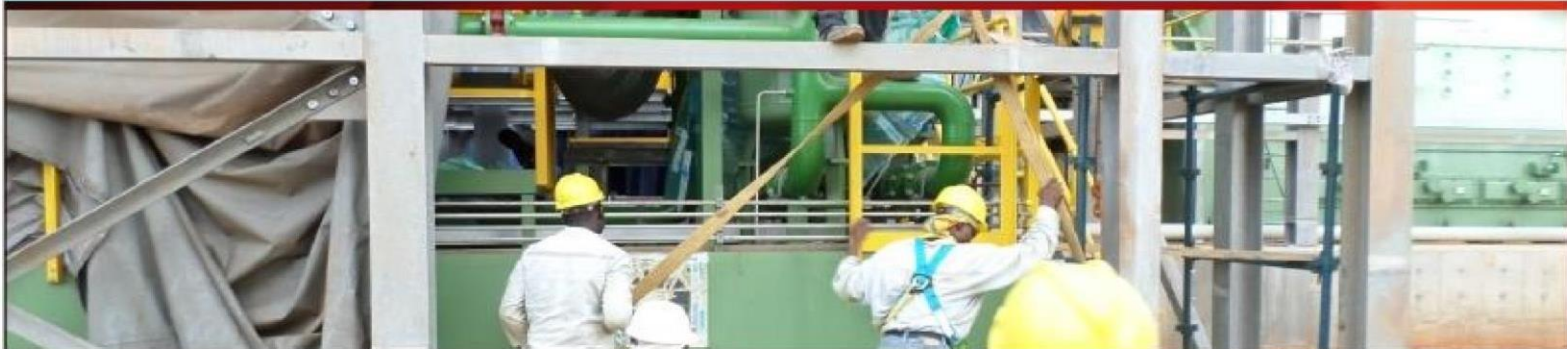
Kpone Thermal Power Project KTPP 1 Installation Of lube oil Piping For the generator, gear box, manifold and diffuser of Gas Turbine 2
