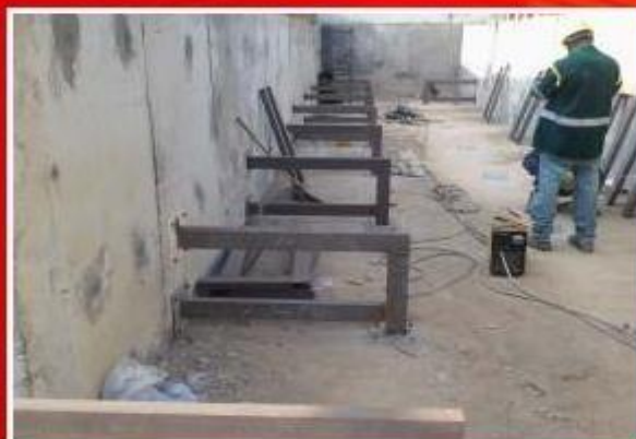
Installation of pipe sleepers and cable racks in the trench
