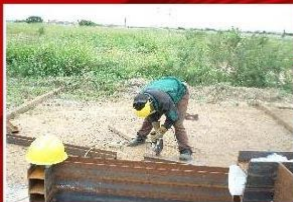
Fabrication of pipe sleepers and cable racks
