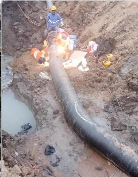
Installation of 16" LNG Pipeline from VRA Gas Interconnecting Facility to the Kpone Power Plant
