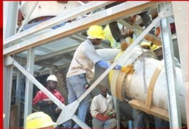
Installation of measurement and blow-off system piping to gas turbine 2
