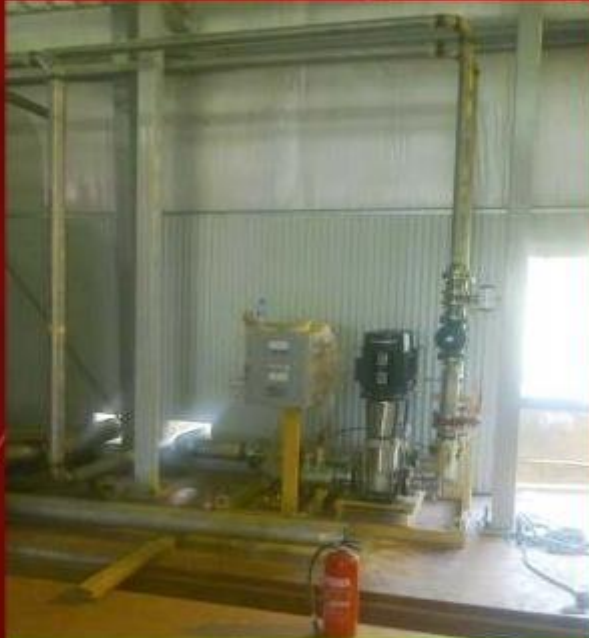
Installation Interconnecting Piping For Forwarding Demineralized Water T3 Project
