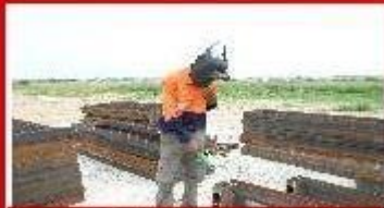
FABRICATION OF SUPPORT FOR CABLE AND PIPE RACKS
