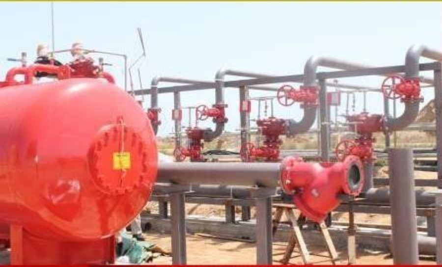
Installation of interconnecting pipes for foam station and the deluge valve assembly
