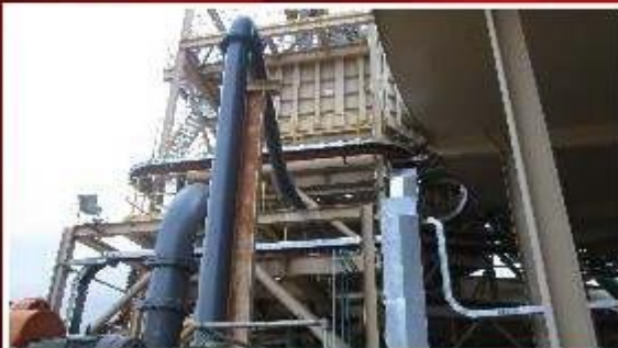
HDPE works for fresh water pump station at Kpone thermal KTPP
