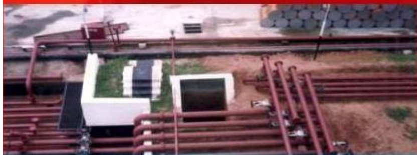
Interconnecting piping at GOIL bulk oil storage facility, Takoradi
