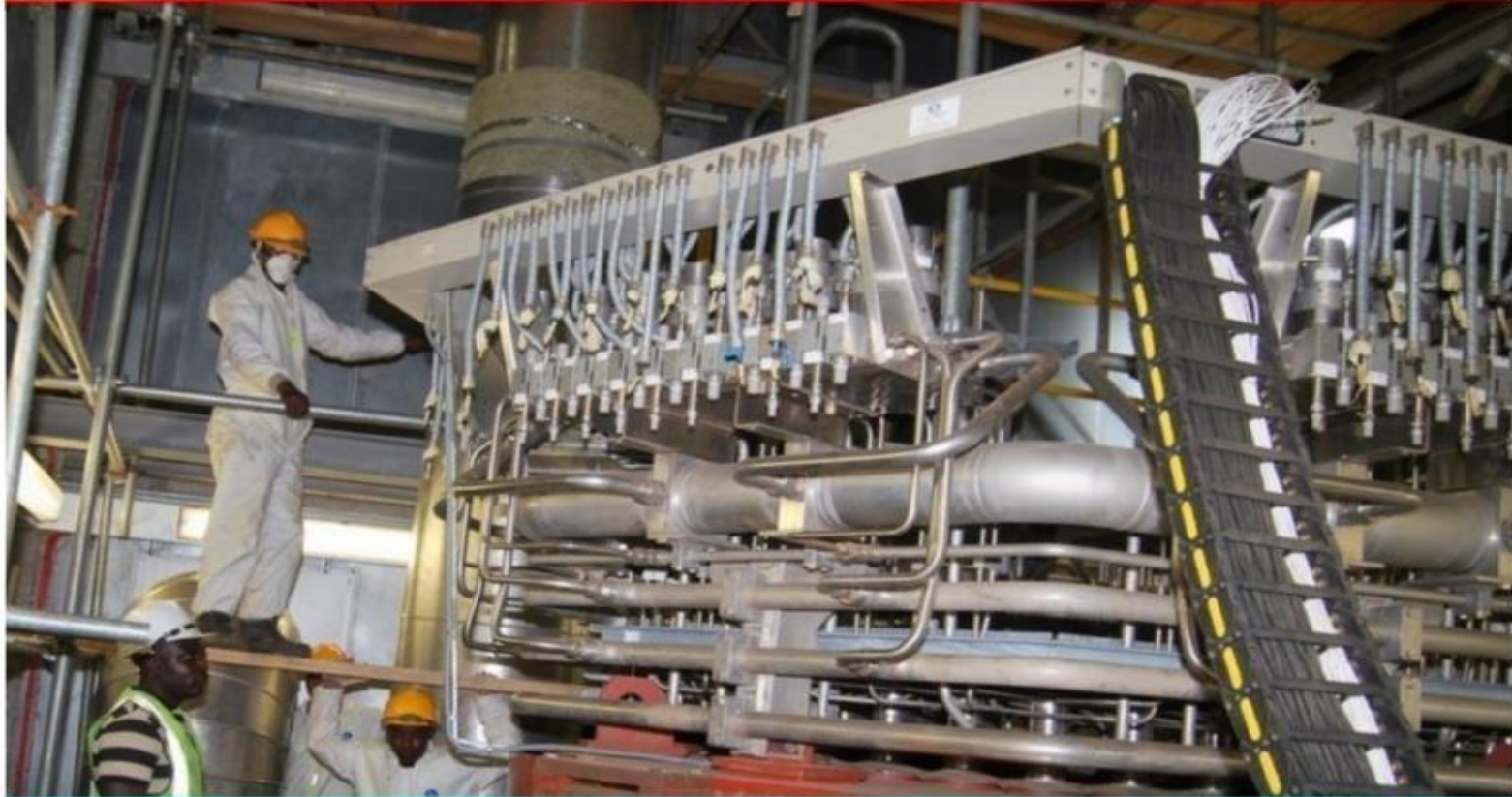
Kpone Thermal Power Project KTPP 1 Installation Of fuel-oil, fuel-gas, nox-water and hydraulic oil Piping to the combustion chamber of Gas Turbine 2
