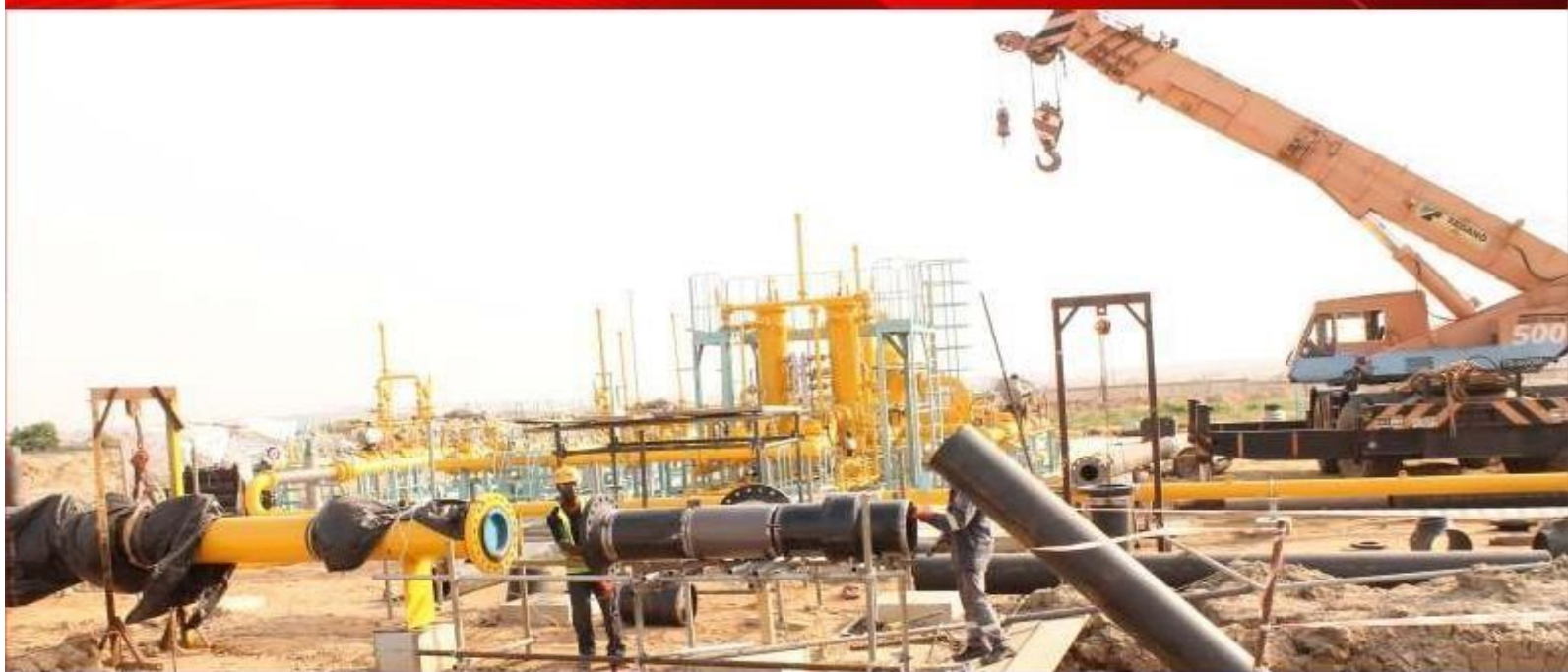
Installation of Interconnecting piping for the LNG receiving, regulation and metering station KIPP
