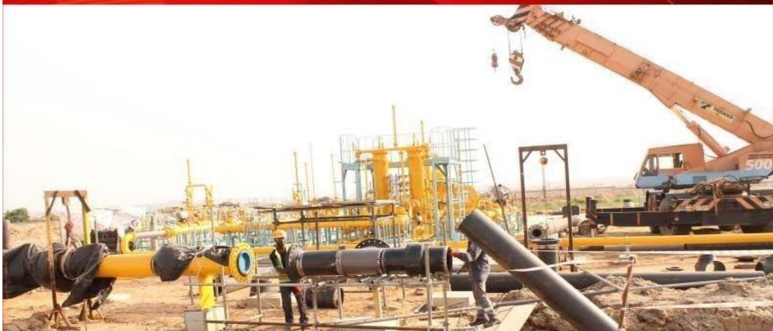
Installation of Interconnecting piping for the LNG receiving, regulation and metering station KTRP
