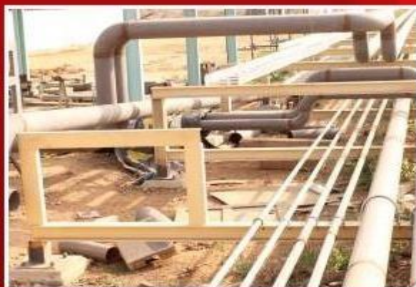
Installation of pipe sleepers and cable racks for balance of plant at KTPP
