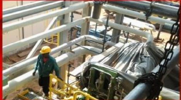
Kpone Thermal Power Project KTPP 1 Installation Of lube oil Piping For the generator, gear box, manifold and diffuser of Gas Turbine 2
