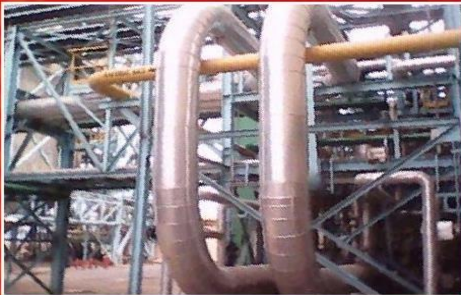
Insulation works at Adamus Mines, Nzema, Ghana
