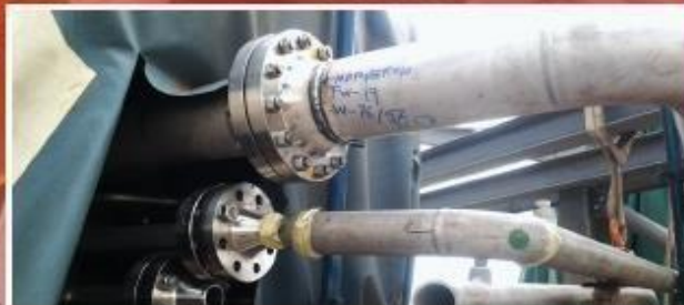
Kpone Thermal Power Project KTPP 1 Installation of fuel-oil, fuel-gas and nox-water piping to the auxiliary block to the combustion chamber of Gas Turbine 2
