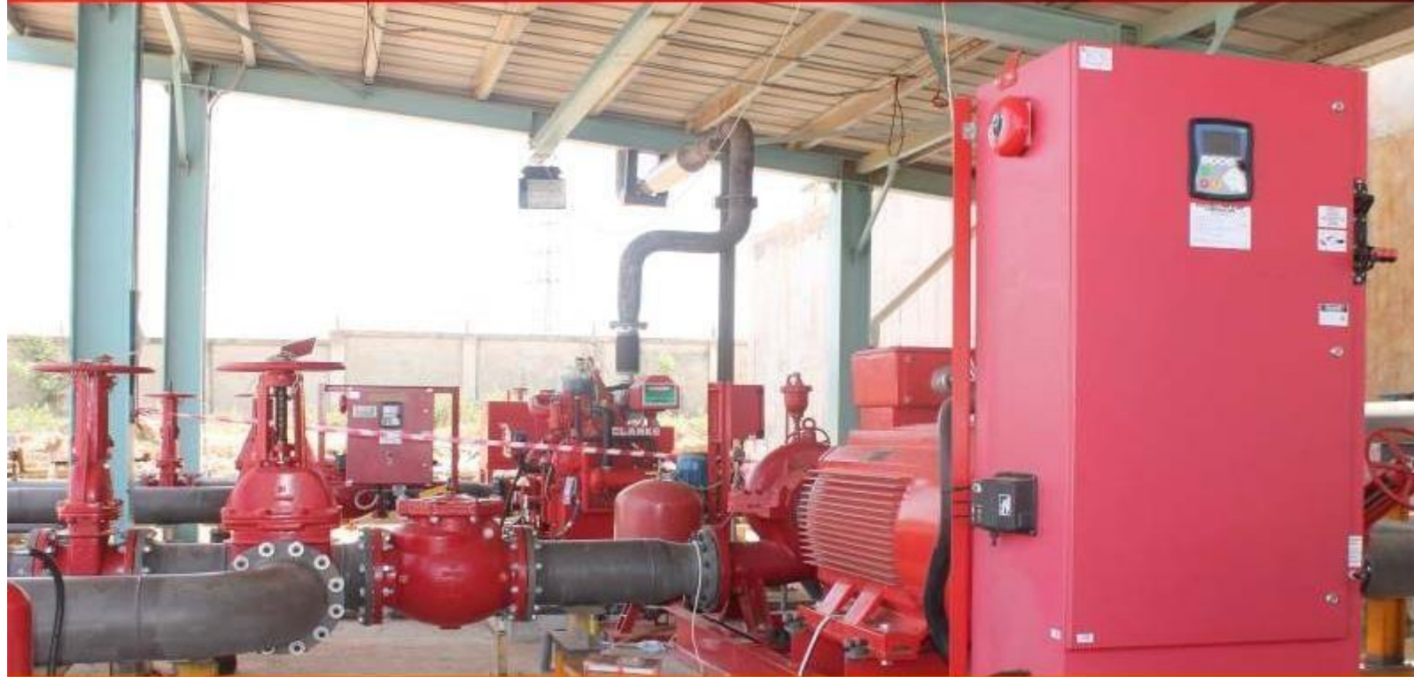
Fire fighting pump station for KTTT
