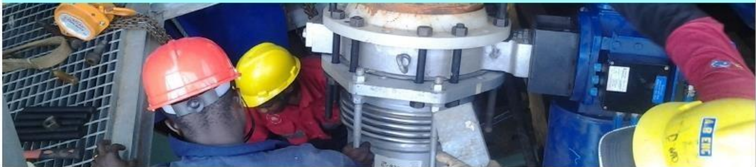
Installation of measurement and blow-off system piping to gas turbine 2
