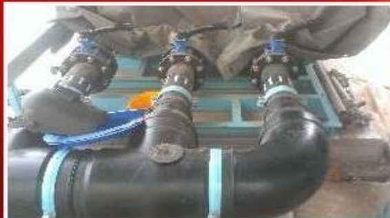
HDPE works for fresh water pump station at Kpone thermal KTPP
