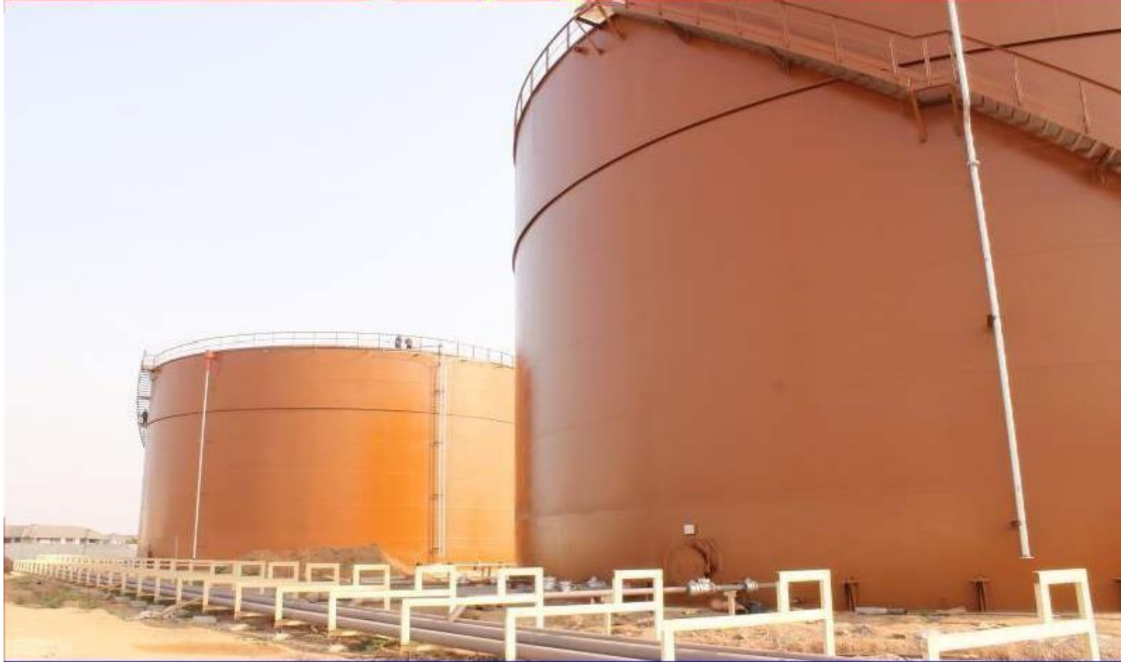
Interconnecting piping for fuel storage tanks of the bulk storage depot GOIL, Takoradi
