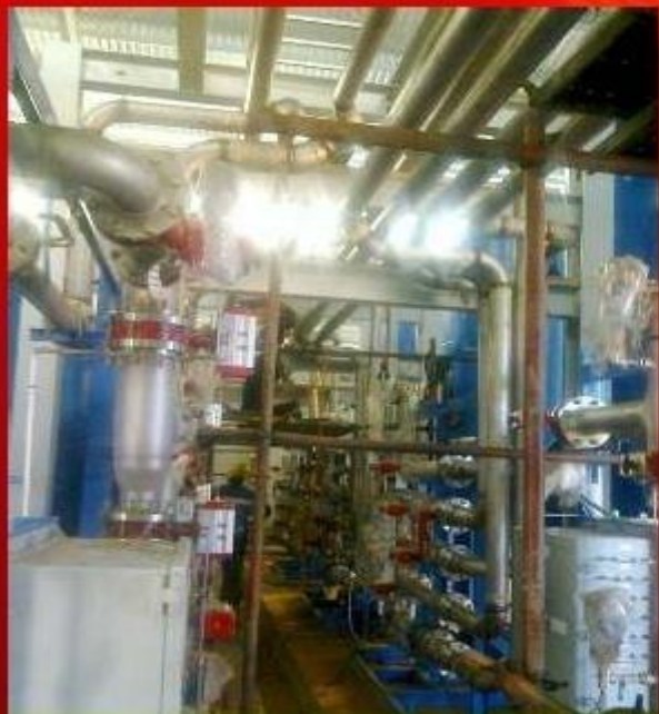
Installation Interconnecting Piping for Anion and Cation Skids
