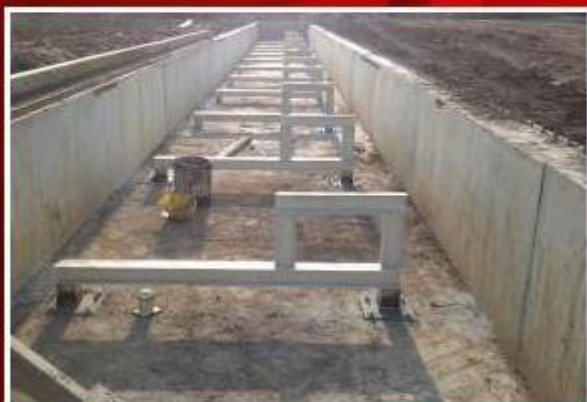
Installation of pipe sleepers and cable racks in the trench
