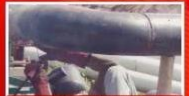
WELDING OF 12" PIPES AT TAKORADI THERMAL POWER PLANT
