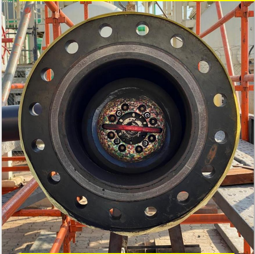
Removal of Smart Pig
