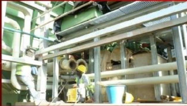
Kpone Thermal Power Project KTPP 1 Installation Of lube oil Piping For the generator, gear box, manifold and diffuser of Gas Turbine 2
