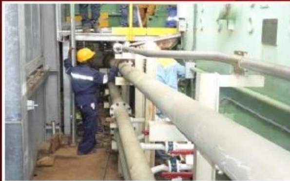
Installation of cooling water piping to the generator of Gas Turbine 2
