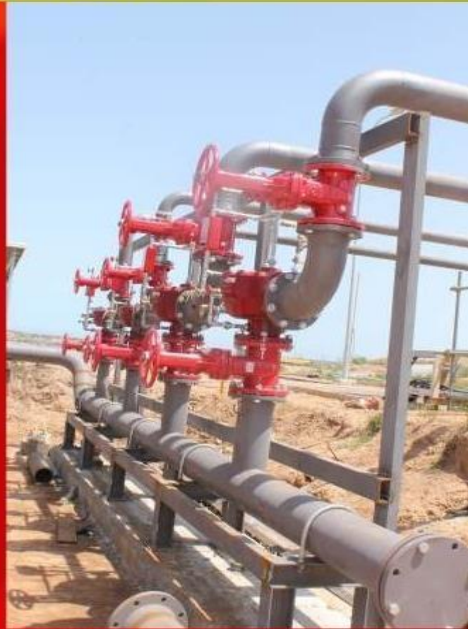
Installation of interconnecting pipes for foam station and the deluge valve assembly
