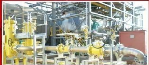
Kpone Thermal Power Project KTPP 1 Installation of fuel-gas piping to fuel-gas skid of Gas Turbine 2
