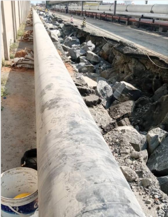
Installation of 16" LNG Pipeline from VRA Gas Interconnecting Facility to the Kpone Power Plant
