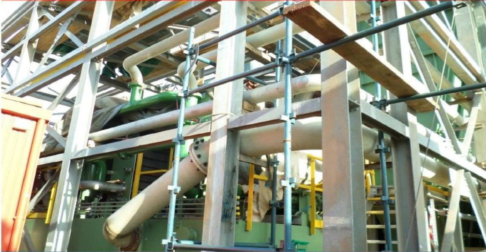
Kpone Thermal Power Project KTPP 1 Installation Of lube oil Piping from auxilliary block to the generator, gear box, manifold and diffuser of Gas Turbine 2
