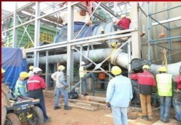
Installation of measurement and blow-off system piping to gas turbine 2
