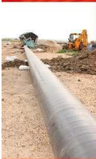
Interconnecting piping for fuel storage tanks of KTPP
