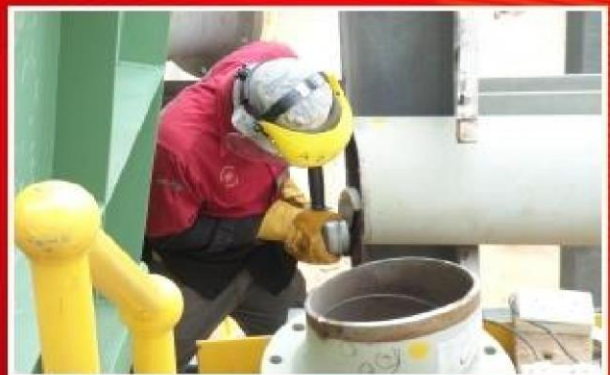
Installation of cooling water piping to the gear box of Gas Turbine 2
