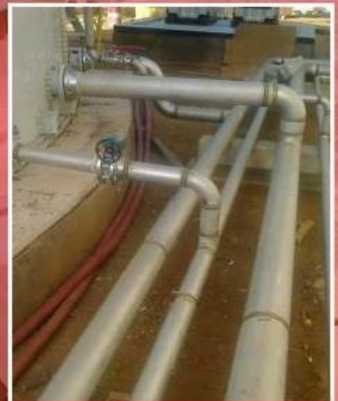
Installation of pipes at the Demineralized waterarea -T3 project VRA-Aboadze
