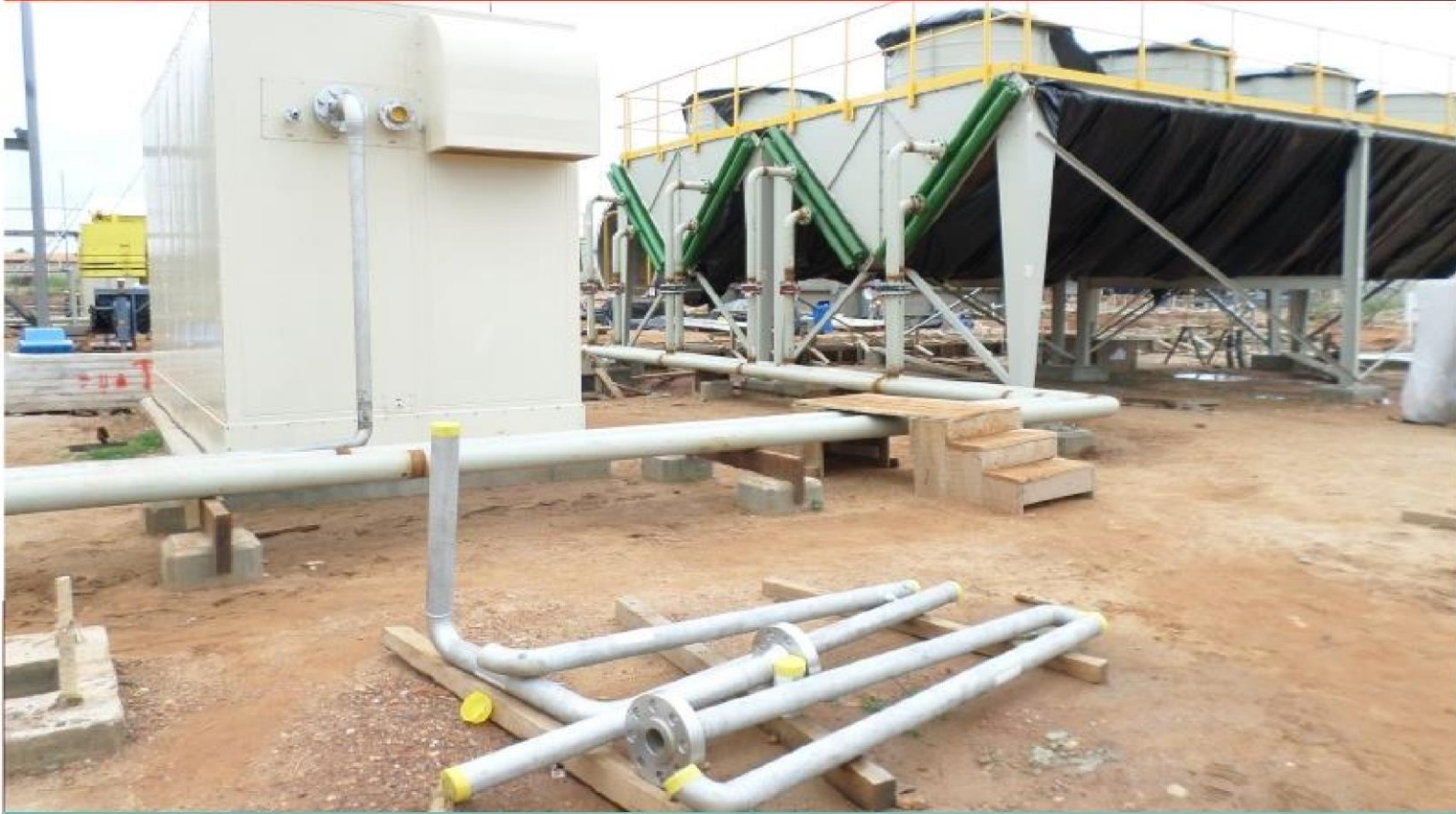
Kpone Thermal Power Project KTPP 1 Installation Of Interconnecting Piping For the cooling tower of Gas Turbine 2
