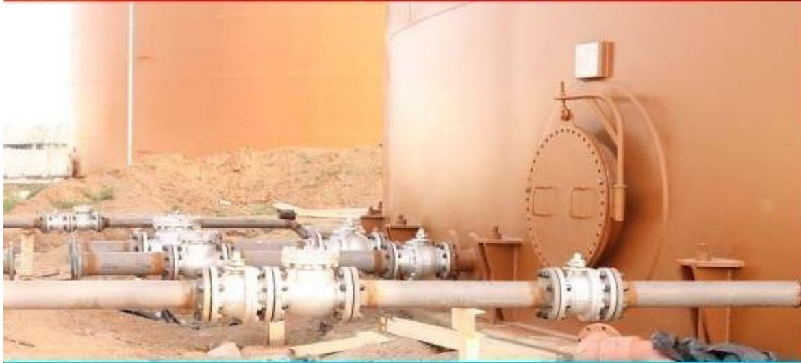
Interconnecting piping for fuel storage tanks of KTPP
