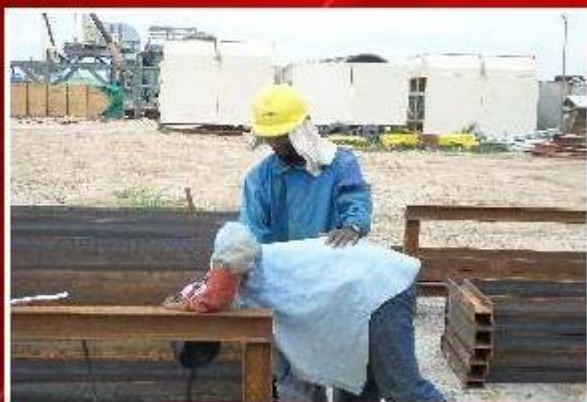
Fabrication of pipe sleepers and cable racks
