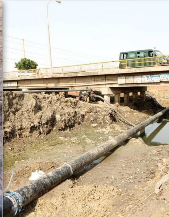
Installation of 16" LNG Pipeline from VRA Gas Interconnecting Facility to the Kpone Power Plant
